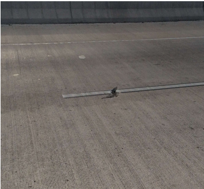
PHOTO 1 Description Spall in the driving surface of span # 3 at centerline.
