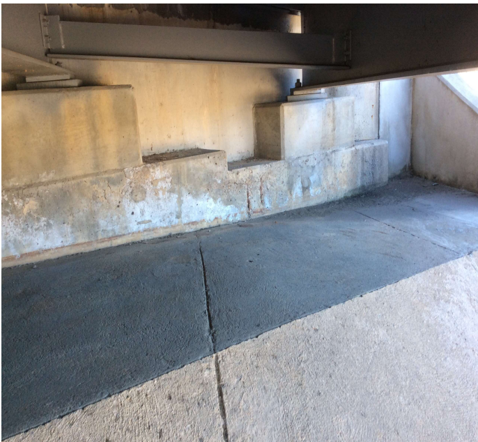
PHOTO 1 Description Bent # 1 left end of the cap spalling with exposed reinforcing steel.
